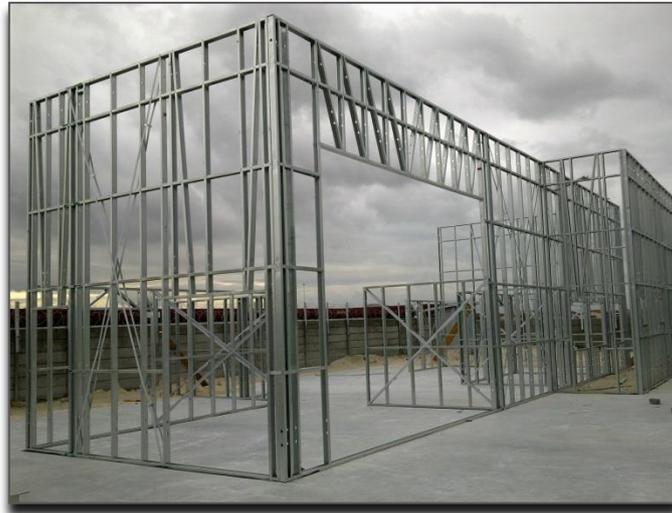
Light Steel Frame is covered with various cladding options that can be plastered to give a traditional brick and mortar or alternative finish according to client or architect specifications. Insulation is placed inside the walls, ensuring superior thermal properties that save electricity while controlling temperatures inside the building.
