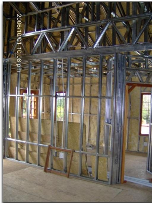
Exterior cladding can consist of a single skin brick wall or fibre cement board, fixed to the wall frames. Services – electricity and plumbing – are installed in the wall cavity created by the light steel frames, as is the insulation material. Gypsum board, fixed to the light steel frame, is typically used for internal wall cladding and ceilings.
